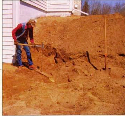
Johnson lays the bottom timbers in the trench, tamps soil beside them to hold them in place, drills a 1/2-in.-dia. hole 2 ft. from each end, and drives a 36-in. length of 1/2-in. rebar through each hole to resist the pressure of soil behind the wall.
